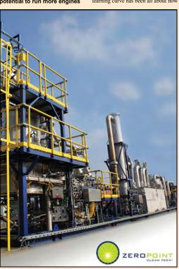
Producing syngas from biomass gasification and then using this gas to generate power using a reciprocating engine is not a new concept, yet it is a technology that has not yet seen widespread commercial application at industrial scale. application at industrial scale. However, US-based technology
